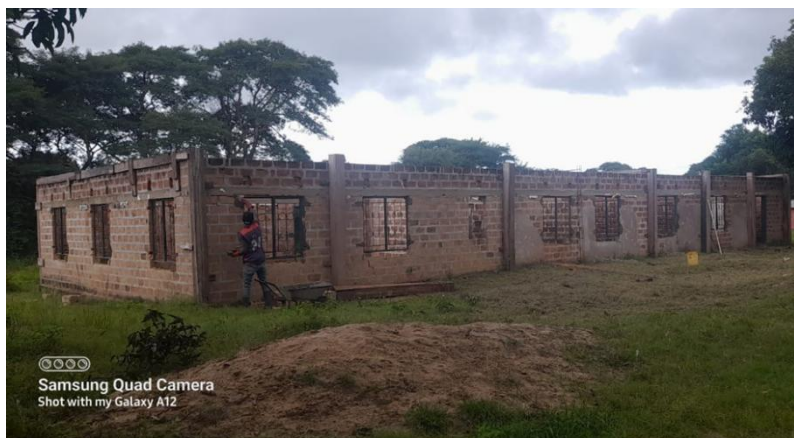
Windows being installed in the girls' dormitory.
